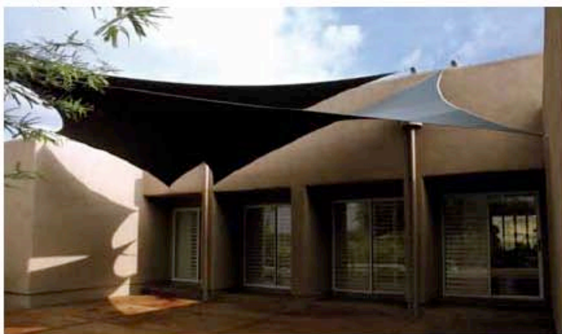
The South patio has two four-point shade canopies that attach to the house at six alternating high and low points to create natural stack venting.
